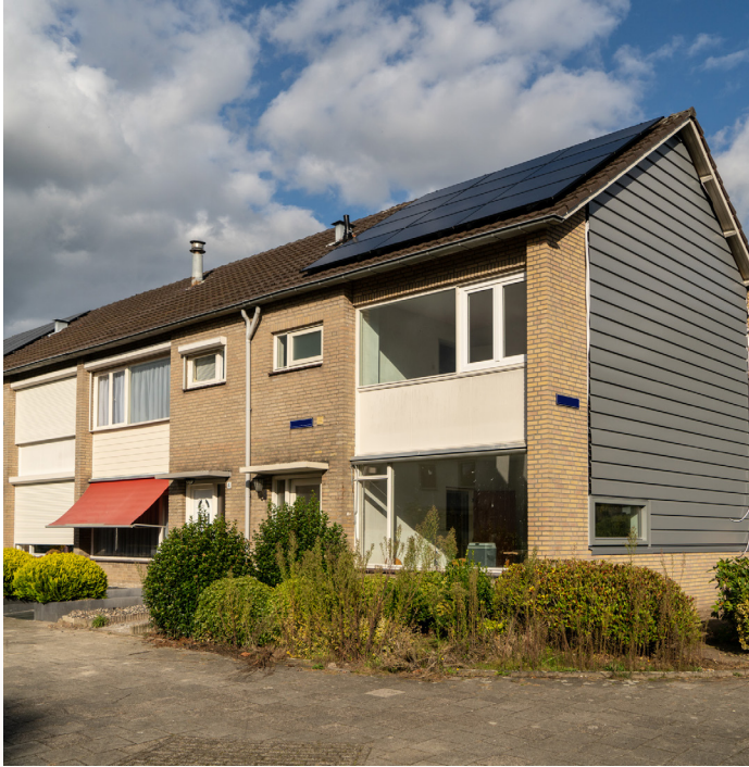
Heat Harvesting panel installed in the site of Eindhoven
