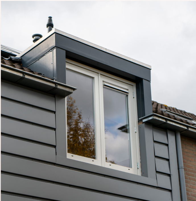
Heat harvesting panel installed on a façade in Helmond
